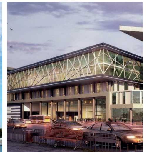
> DEWA (Dubai Electricity & Water Authority) Office Building, Al Ruwaihah, Dubai
